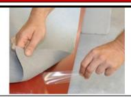
**9.3** apply the membrane and remove the tapes paper cover
