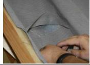
**9.9 - 9.10** The membrane overlaps of the valley stripe connect with tape JUTADACH SP 38
