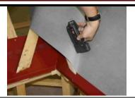
**9.5** fix the membrane with staples to a side of valley counter batten
